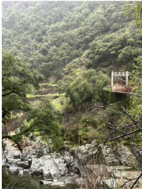
Nothing to the south of the bridge will remain including historic rock walls.
