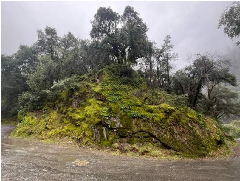
The spine of this ridge will be destroyed, massive cut and fill.
